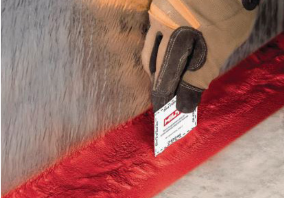
Figure 5.2 Example of visual inspection
