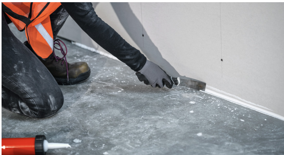
Figure 4.2 Example of linear firestop joints
