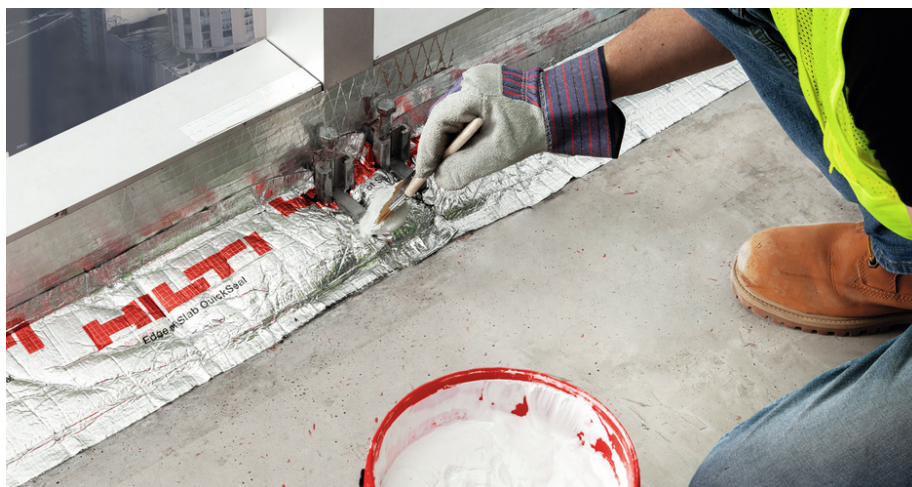
Figure 2.10 Perimeter firestop joints
