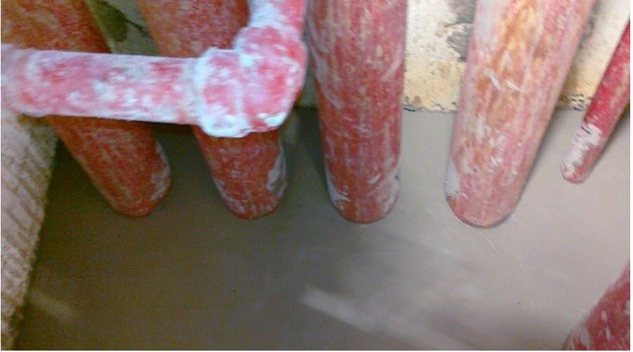
Figure 2.8 Firestop for sealing shafts
