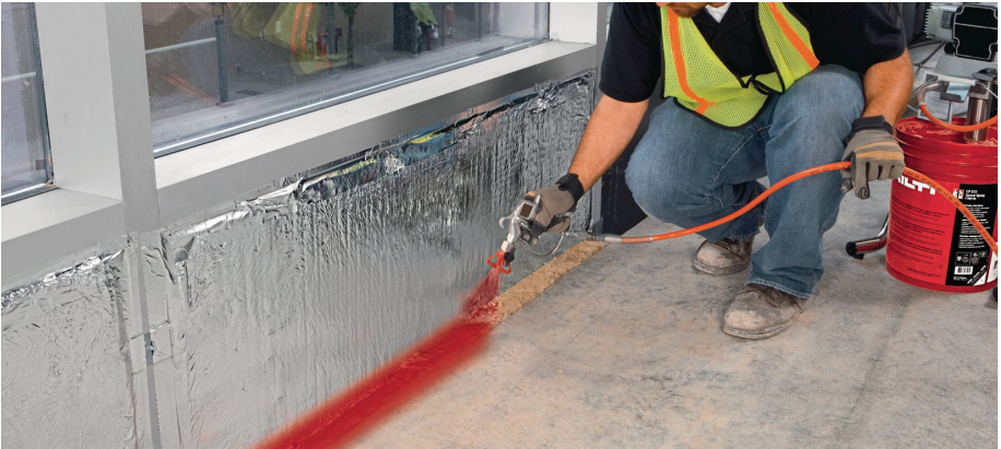
Figure 4.1 Perimeter firestop joints
