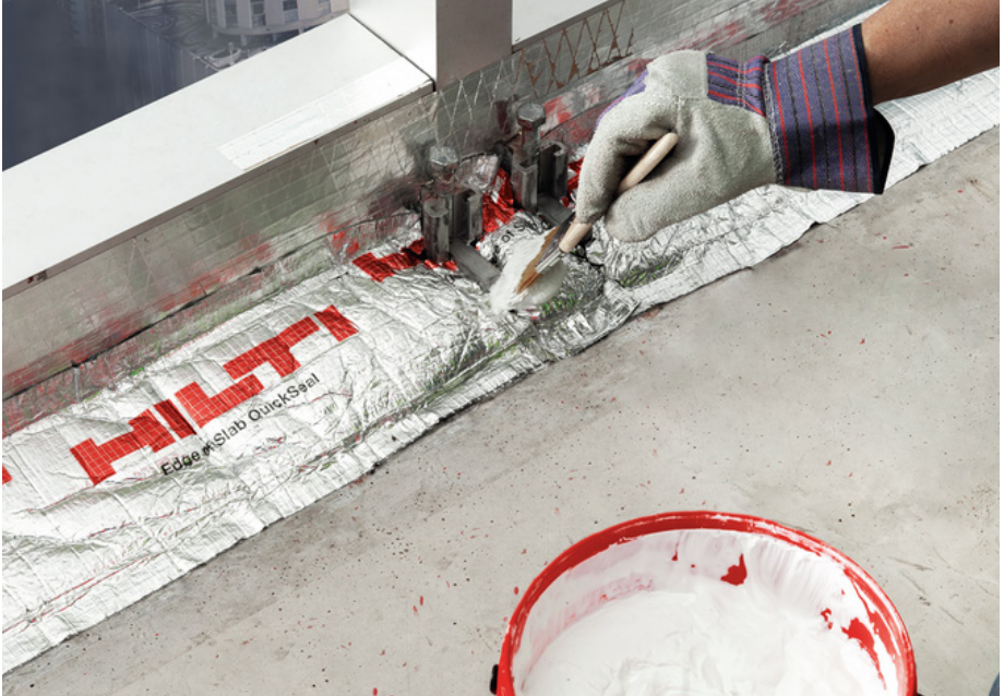
Figure 4.3 Example of perimeter firestop joints
